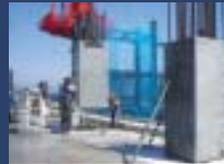
PCa units manufactured in factories in advance are used for the columns, beams, walls and floors of building frames. The only work required at the building site is to assemble the parts; it is possible to omit formwork, reinforcement work, etc., which means that onsite tasks can be made more efficient and construction can be completed more rapidly.
