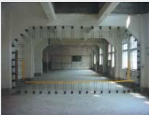
We have been developing the steel tube cotter method into a quakeproof reinforcement method and acquired an architectural technology certificate for it through examination by the General Building Research Corporation of Japan. Now that we have obtained a performance guarantee by a third-party organization, we can omit explanation to individual examination agencies when we use this method in quakeproof reinforcement works.
