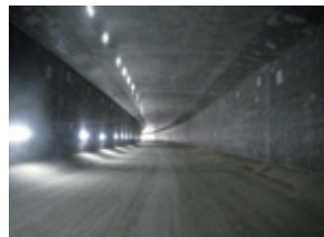
Shichiyama Bypass Fukube Sakyu Tunnel Location: Tottori, Japan Client: Chugoku Regional Development Bureau of the Ministry of Land, Infrastructure, Transport and Tourism
