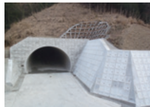
Chubu Odan Expressway Daigoyama Tunnel Location: Minobu-cho, Yamanashi, Japan Client: Kanto Regional Development Bureau of the Ministry of Land, Infrastructure, Transport and Tourism
