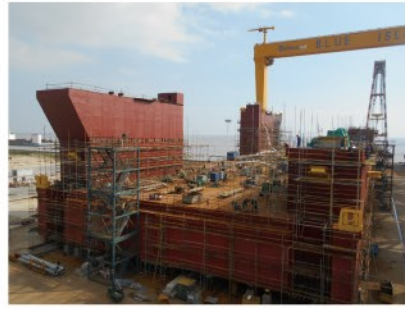
02 Island part construction
