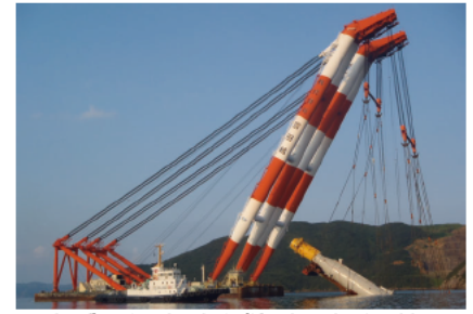
3. The floating body is lifted and raised by a large floating crane, and floated on the sea.
