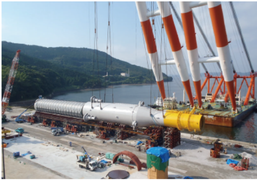
1. Steel upper floating body manufactured in a plant is connected with concrete-made lower floating body at the quay to complete the hybrid spar-type floating body.
