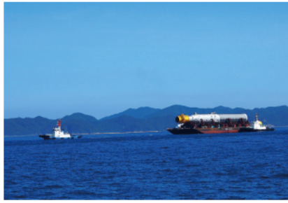
2. The floating body (hybrid spar type) is loaded onto a salvage barge and transported to the assembly site in the sea north of Kabashima.
