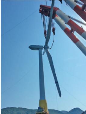
1. Steel upper floating body manufactured in a plant is connected with concrete-made lower floating body at the quay to complete the hybrid spar-type floating body.
