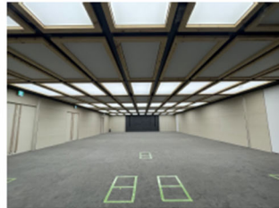
(Wooden frames for ceiling lighting)
