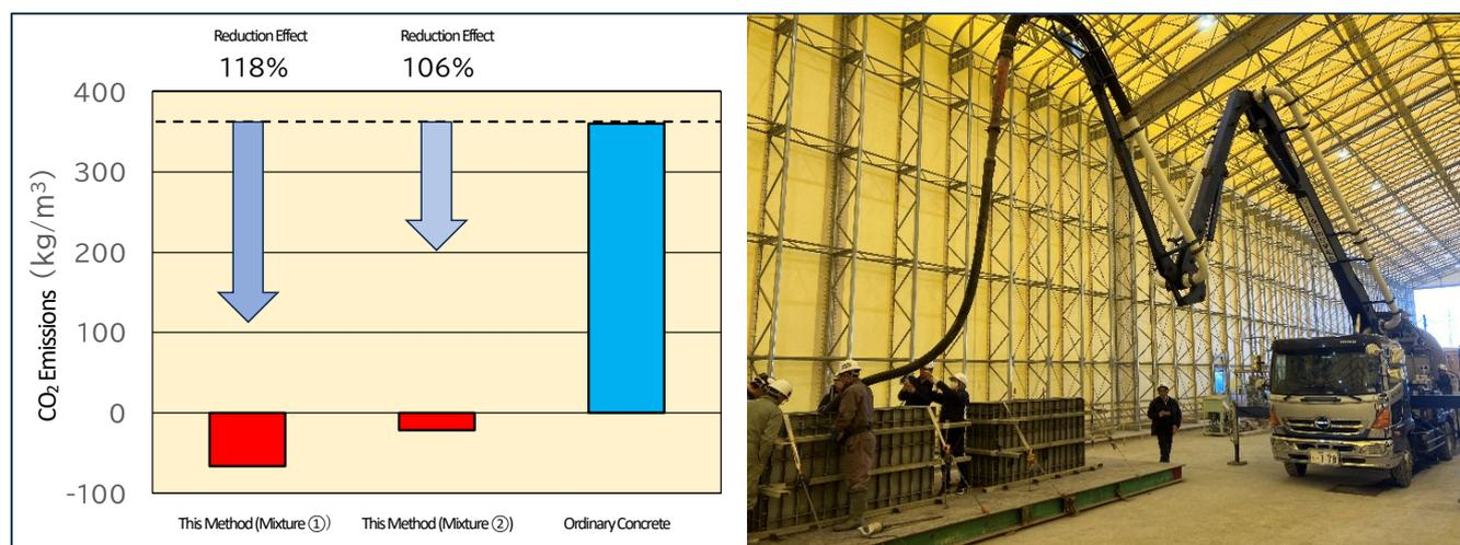
Figure 1 CO<sub>2</sub> Reduction Effect of Carbon-negative concrete ※2 and Photo showing pouring concrete
