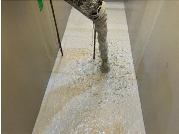
Picture 1: Outlet pouring Carbon Negative concrete
