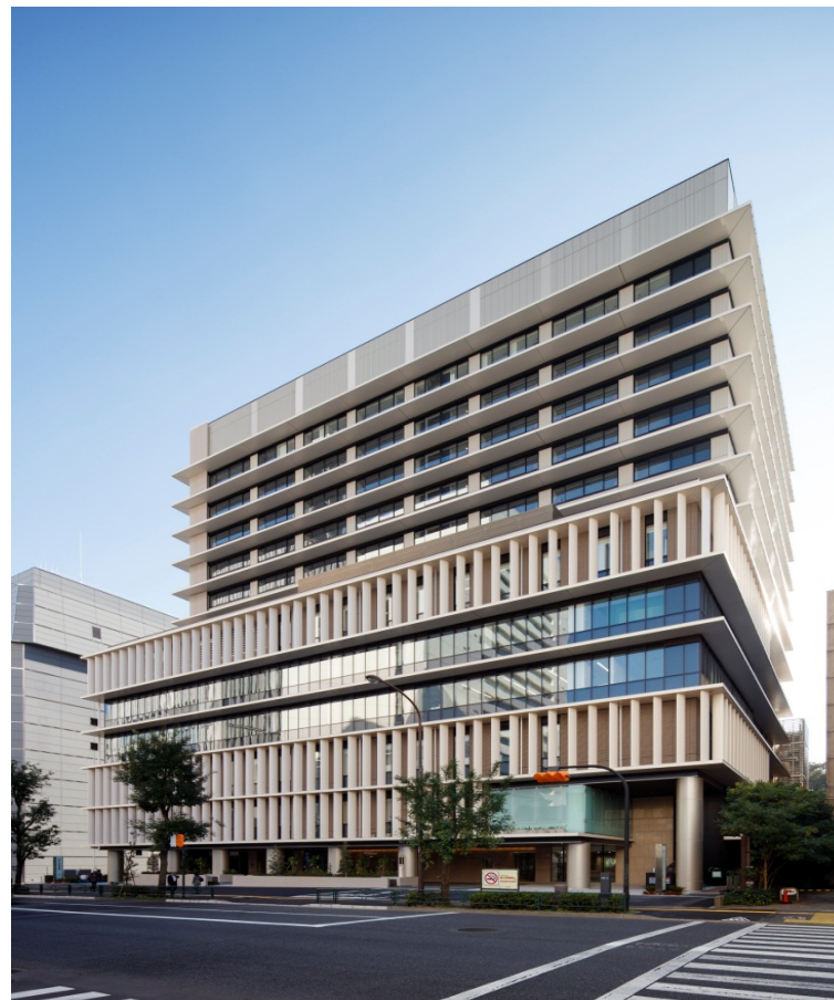
Kudanzaka Hospital complex building work, Federation of National Public Service Personnel Mutual Aid Associations
