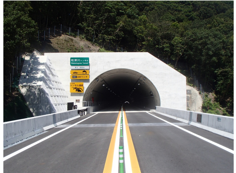
Kinki Expressway Kisei Line Wabukagawa Tunnel, Ministry of Land, Infrastructure, Transport and Tourism, Kinki Regional Development Bureau
