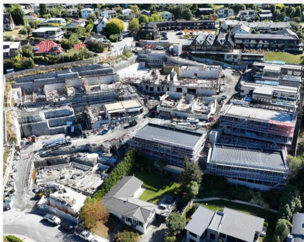
Construction status: overall view
