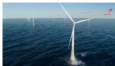
Hywind Tampen (88MW, Operational from 2022)
