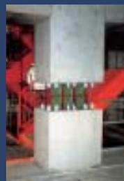
The RC studs are constructed with special embedded steel plating, which has the flexibility to be moderately deformed in earthquakes. This allows not only a reduction in the effect of earthquake tremors, but also the minimization of damage to the building.
