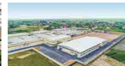
PHO YEN FACTORY WORKER'S CANTEEN, CHANGING ROOM, PARKING LOT[ベトナム] 発注者：MANI HANOI CO., LTD. (ベトナム戸田建設(有)施工)
