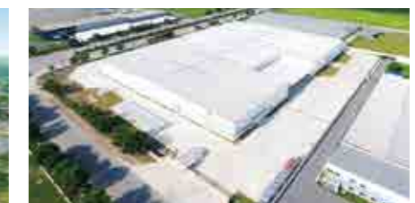
NIPPON KONPO VIETNAM WAREHOUSE LEASING SERVICE PROJECT[ベトナム] 発注者：NIPPON KONPO VIETNAM REAL ESTATE CO., LTD. (ベトナム戸田建設(有)施工)
